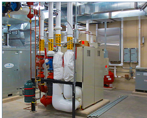
Nebraska Army National Guard Readiness Center, Mead, NE • Geothermal loopfield system
