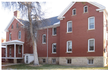
Renovate Building B3, Veterans Affairs Medical Center, Sheridan, WY • New fire sprinkler system
