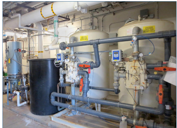
Indian Health Services, Winnebago, NE • Central utility plant conversion study
